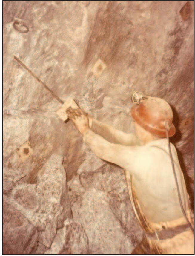
Miner Franklin Kramer inserting a rock bolt into the bore hole.
