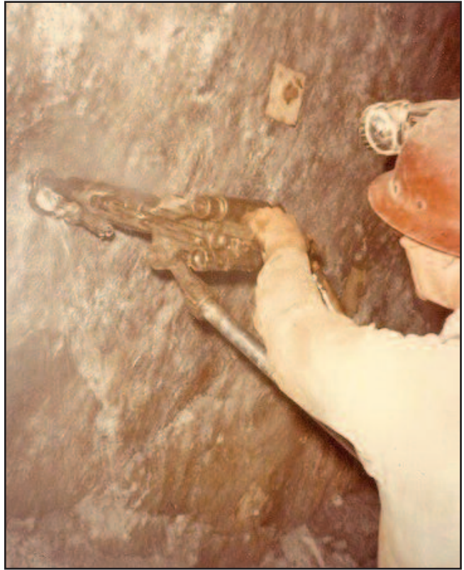
Miner Franklin Kramer drilling a hole for the rock bolt.
