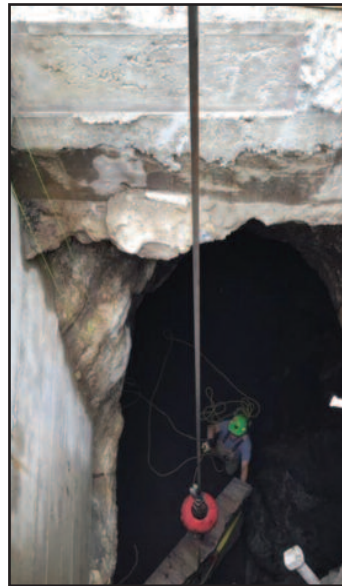
John Gumbs, receiving the slab in the stope.
