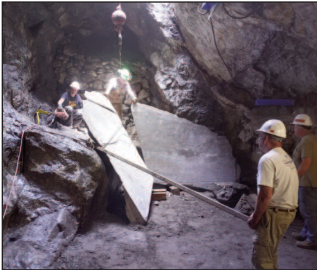
Bill Kroth, adjusting the placement of the second slab.
