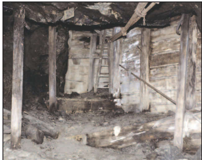
This is the base of the man-way up into the 800 stope off the 340 foot level. These fences were built to hold back the fill rock. There were hundreds of these fences throughout the mine, some much bigger than this one.
