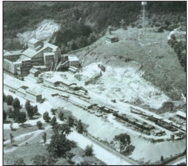
Rare late 1930s era aerial view of Sterling Hill. Note the Great Sterling Mill complex, the new office building, the water tower on the hill, and the ten small ore bins near the south garage area where the ore cars were loaded. Also note the line of empty gondola cars being backed in over the trestle, to be loaded.
