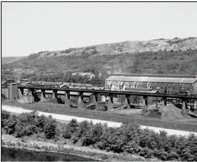
1950s era photo of the Palmerton Processing Plant. Trains came in from the left (west), were backed onto the elevated tracks in front of the plant, where they were unloaded, and the ore was brought by bucket loader into the plant.
