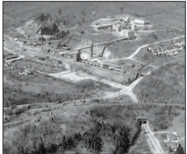
1960s era aerial photo of Sterling Hill. Wow, what a difference! Note that the entire Great Sterling Mill complex has been removed; and the new upper complex buildings, conveyor, and ore bins have been constructed. The lower headframe remains as well as the water tower. The railroad tracks over the backwards tunnel have been abandoned and removed.
